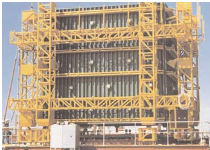
High speed railroad structural column
